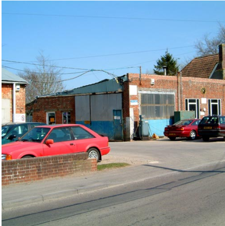
Functional but unattractive. The buildings of the former Old Forge Garage have seen better days and their prominent position in the High Street makes this visually one of the least attractive parts of the village.
