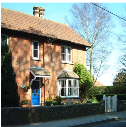
Yew Tree House is a particularly good and unspoilt example of Edwardian architecture. There are a number of unlisted historic buildings in Worton and these make up a significant part of the Conservation Area
